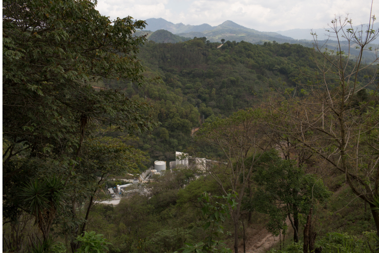
(Entry point to Tahoe Resources' second tunnel, down the mountain side from La Cuchilla community. San Rafael Las Flores municipality, Guatemala. Photo, May 22, 2016, by James Rodriguez, www.mimundo.org )
